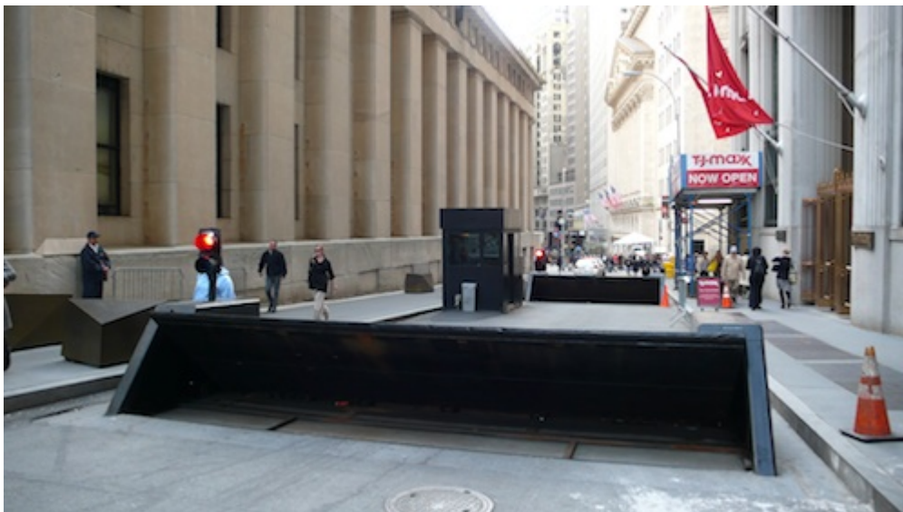
Photo 4 : barrages anti-intrusion protégeant le New York Stock Exchange © J.-Ch. Gay, 2012.
