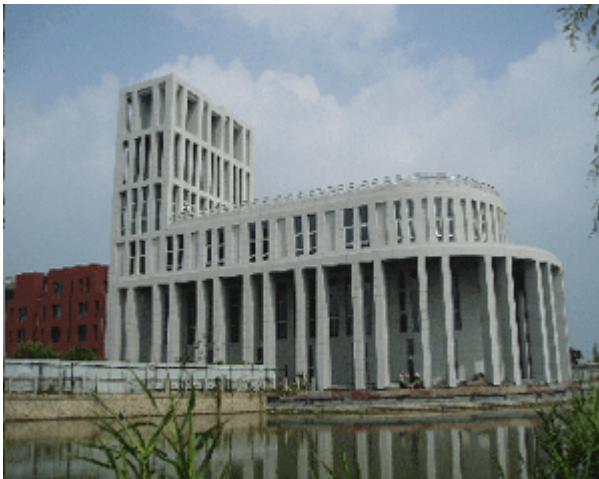
Fig. 9 : Anting Church (under construction).
