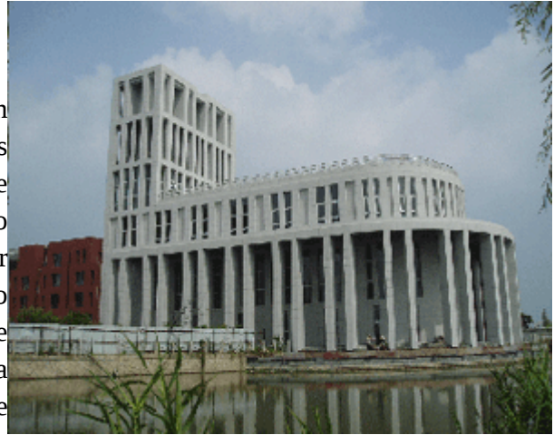
Fig. 9 : Anting Church (under construction).
