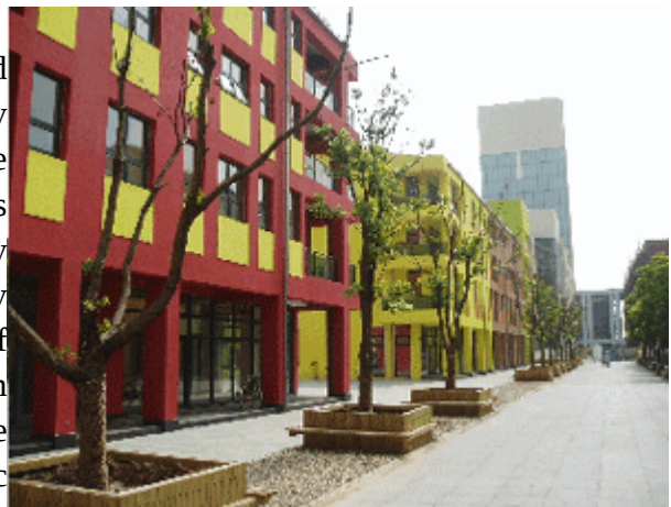
Fig. 3 : Residential buildings with commercial ground floor use.
